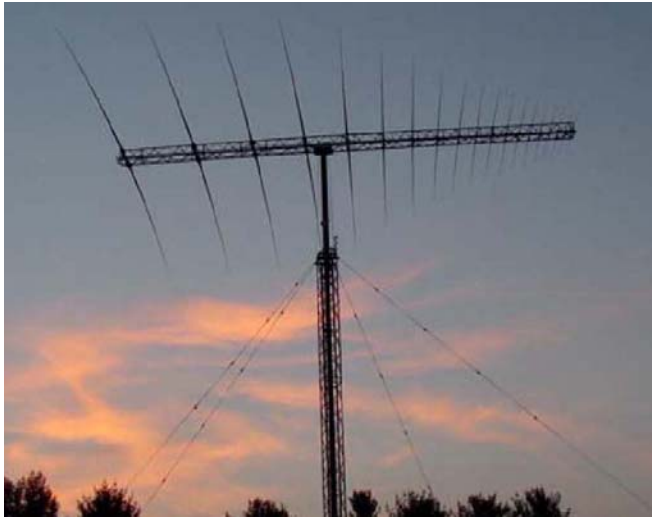
LP1001CA on 3002FA Guyed Tower
